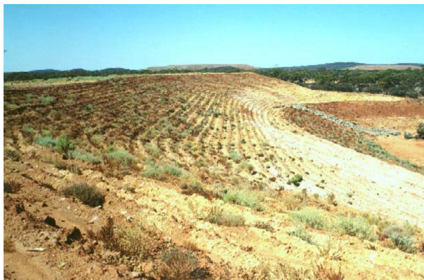
Figure 27. A batter slope that has been contour ripped to produce “bank and trough” physical resource regulating means. There are no
